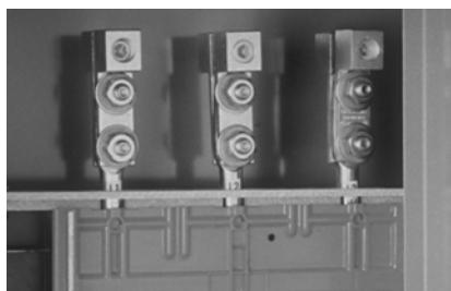
The Bulletin 2191M and 2191F are line lug compartments that provide a lug connection for incoming lines (2191M) to distribute power to the motor control center or for outgoing cables (2191F) to feed power from the MCC to an external load. These line lug compartments are available with ratings from 300 to 2000A. Optional mechanical or crimp lugs can be supplied with the lug compartments.
