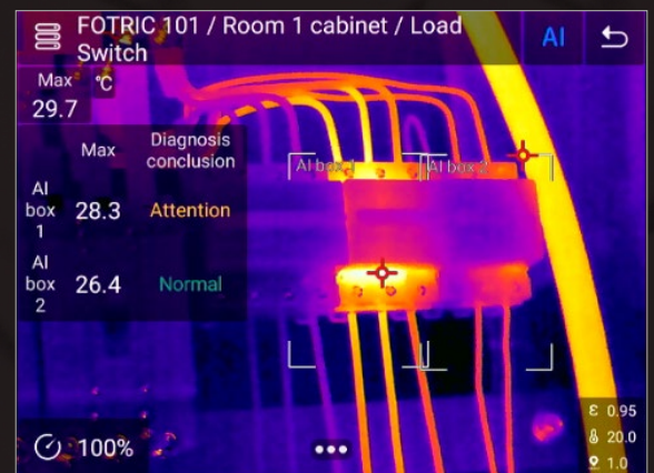
NaviPdM on-device ROI-based alarms
